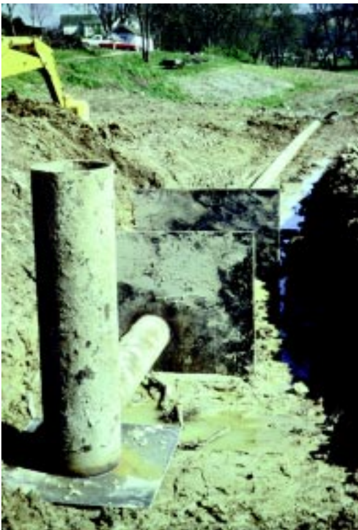
Figure 22 Drop-inlet pipe spillway with antiseep collar
