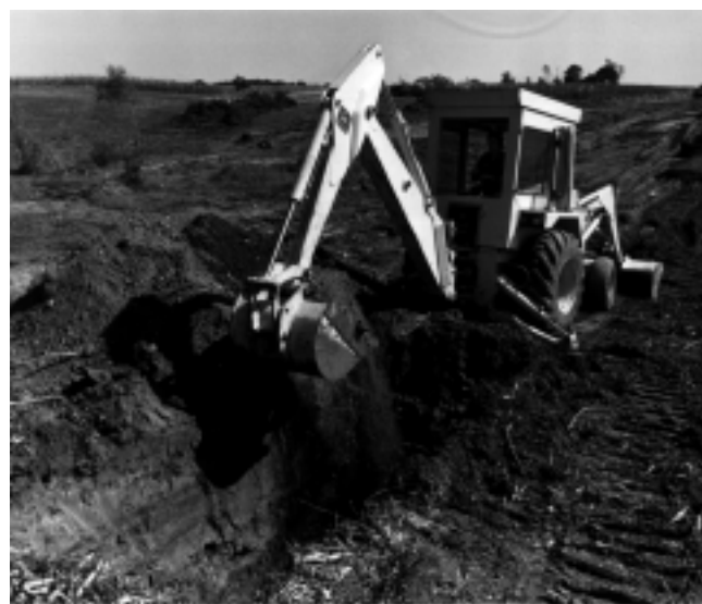
Figure 27 A core trench is cut on the centerline of a dam
